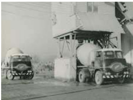
M1 Motorway, Hathern, 1963
