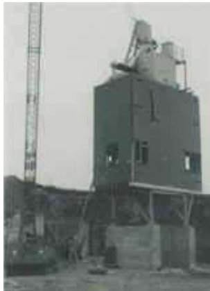
Plant erection nearly done
