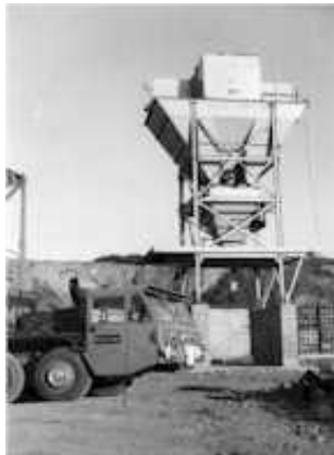
Plant erection continued
