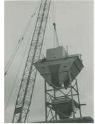
Plant erection continued
