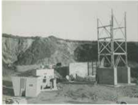
Start of plant erection sequence, 1964
