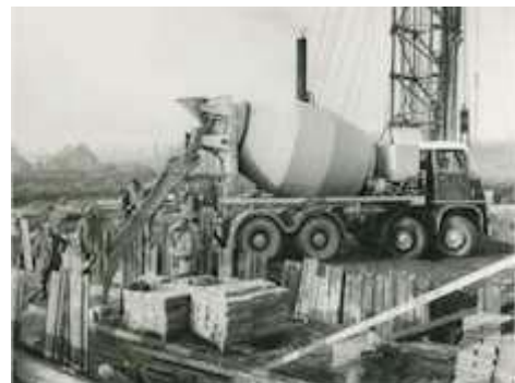
Pouring into bridge foundations
